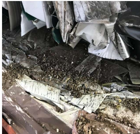
Dirt and Debris
