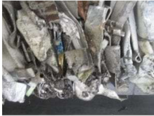
Dirt and Debris
